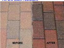
The selection of a sealer will depend on certain criteria. For example, if the pavement to be sealed is around a pool, then a non film-forming sealer that has no impact on slip and skid resistance would be best. If distinct colors are important, then a color enhancing sealer will help best to make the colors stand out. Or you may prefer a natural or an invisible sealer to preserve the natural look of the paver colors.
